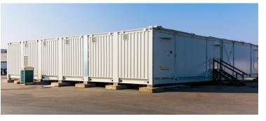
technologies (including room cooling, and SmartAisle containment and control), as well as advanced Lithium Ion batteries for reduced operational expenses. Designed to accommodate ocean shipment, the facility was prefabricated, integrated, and tested in Vertiv's European facility. It was then disassembled into 12 shippable units, packed for transport, and made the journey to South Africa, where it was reassembled on site and ready for testing in under six weeks.
